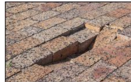
Loose bricks, tiles, paving should be repaired immediately or at least cordoned off to prevent loss or injury
