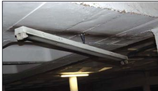
Obvious dangers in basement areas, loose fittings etc. could hurt someone or cause damage to property or vehicles. The insurer would surely not be expected to honour claims where trustees are not taking reasonable care, or precautions to prevent loss
