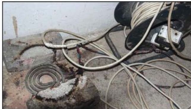
Dangerous electrical connections being used by body corporate employees on common areas - this aspect must be checked
