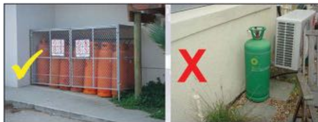
Gas bottles should be stored correctly and safely
