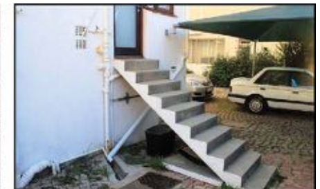
Slopes and stairways should have handrails per national building regulations
